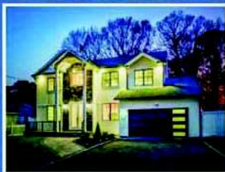
West Hempstead New Construction
